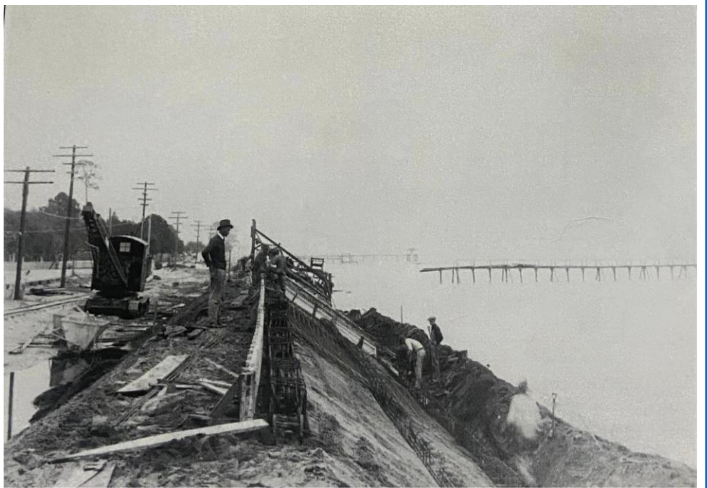
Seawall construction began in the 1920s; completed in 1926
