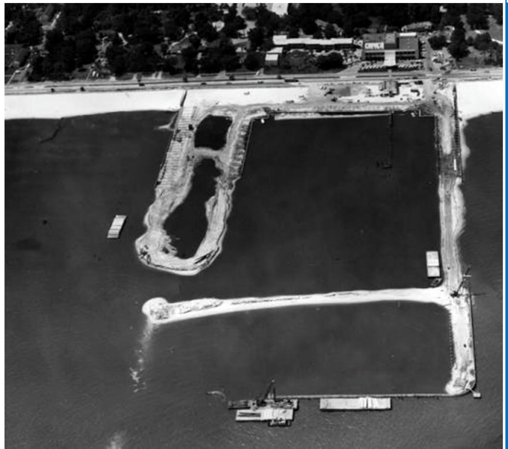
Aerial, Biloxi, 1963, Broadwater Beach Hotel Marina construction in process. Later, a 10 feet deep channel 4,250 feet long was dredged to provide landfill for the marina's land areas (Thanks to Randy Randazzo)
