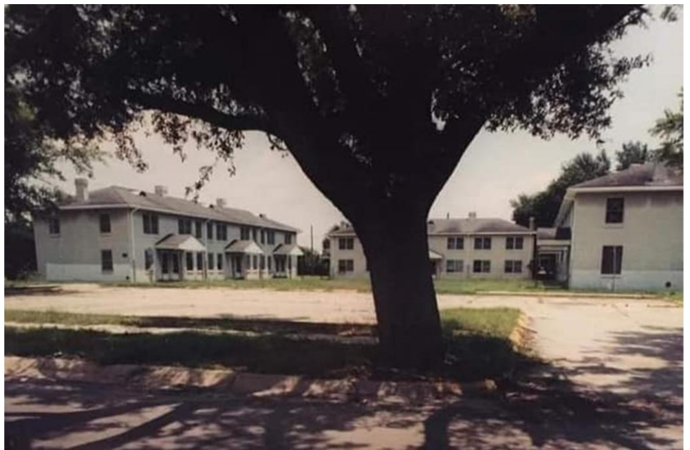
East End Homes, near Howard II Elementary School (Maple & Howard), Biloxi, date unknown (Thanks to Billy Carroll)
