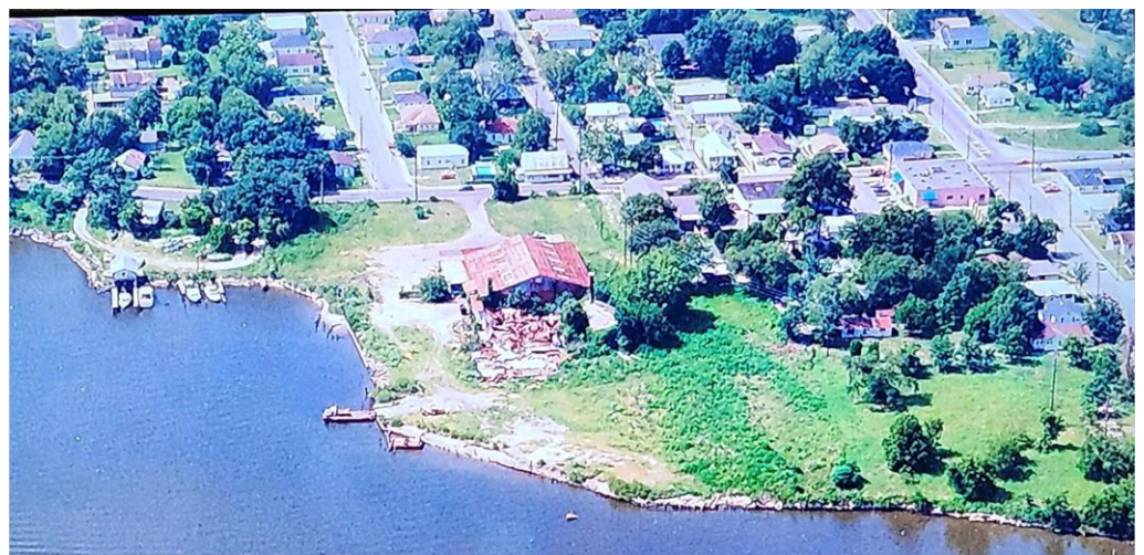
Aerial view, pre-casino, where the IP casino is now located. Caillavet Street is on the right, running north-south; Bayview Avenue is running east-west, Biloxi, date unknown
