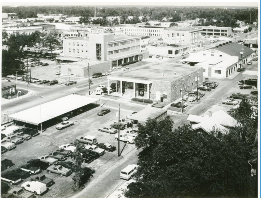
View of Main Street, Biloxi, looking north shows several buildings that are still there such as the Post Office and Masonic Lodge. Dee's Chevrolet (center) and other buildings are not, date unknown
