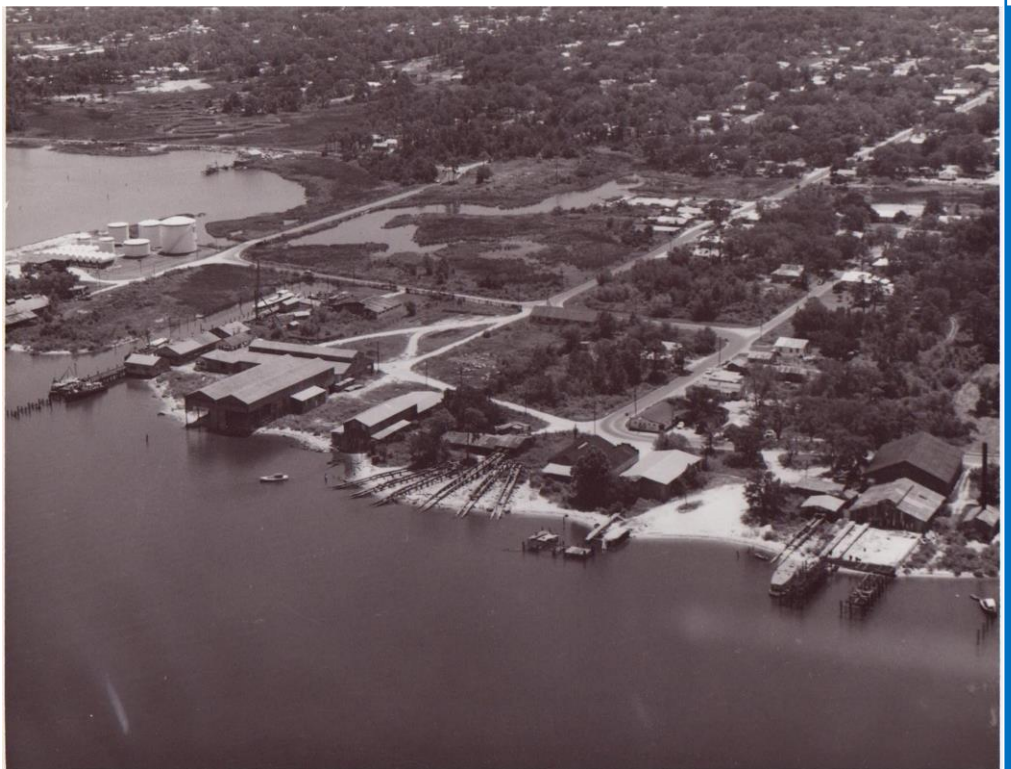
Aerial, Biloxi Bay, Munro Oil (center, left) and boat works, pre-Katrina, no date
