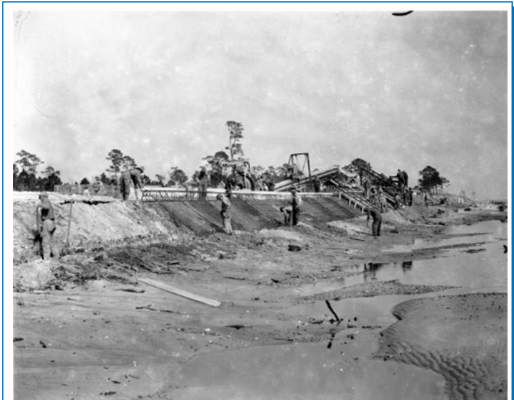
Seawall construction, before the sand beach, Biloxi, no date (Randazzo Collection MDAH)
