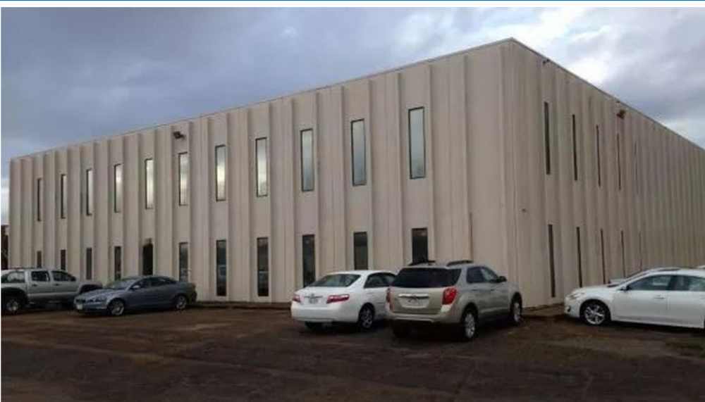
Biloxi's Federal Courthouse, between Howard Ave. and Martin Luther King, Jr. Boulevard; demolished in April, 2018, to make way for Community Bank, now completed, at the northeast corner of Howard Ave. & Main St.
