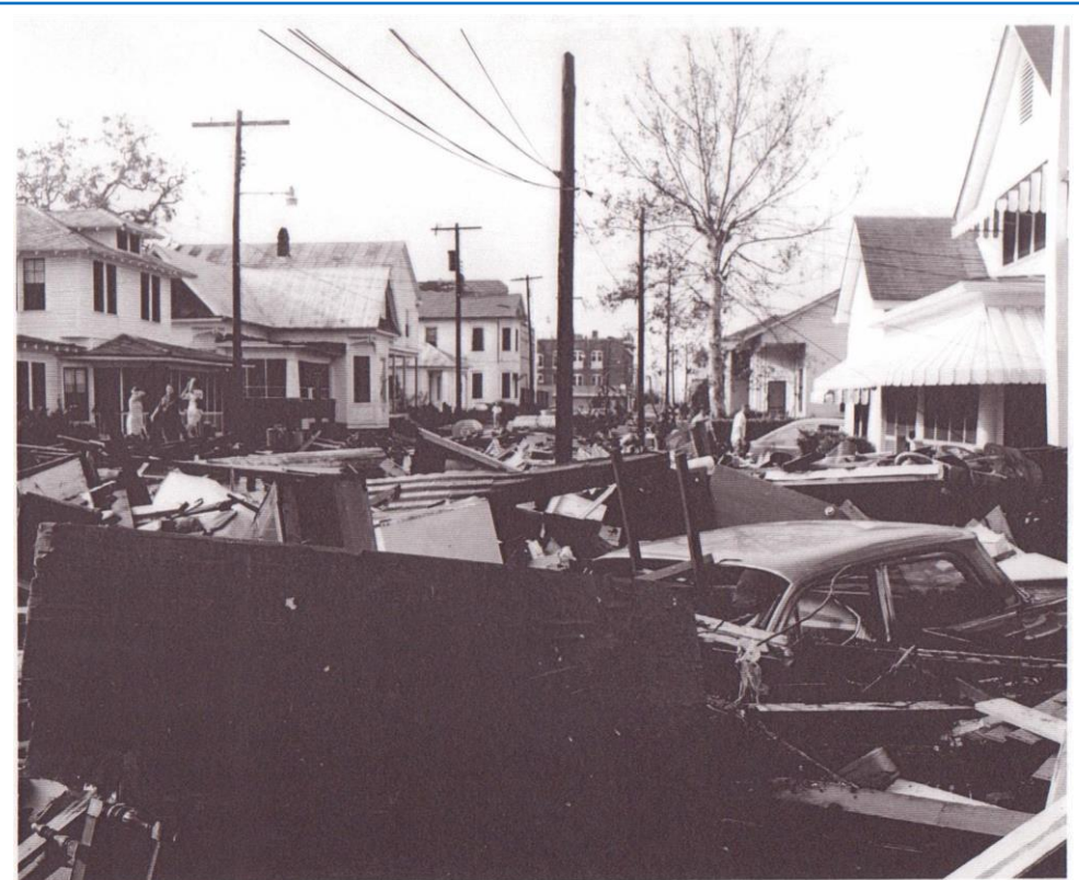
Looking west down Howard Avenue after Hurricane Camille, 1969. I believe that brick building in the center/background is the Masonic Temple on the southwest corner of Howard Avenue & Main Street.
