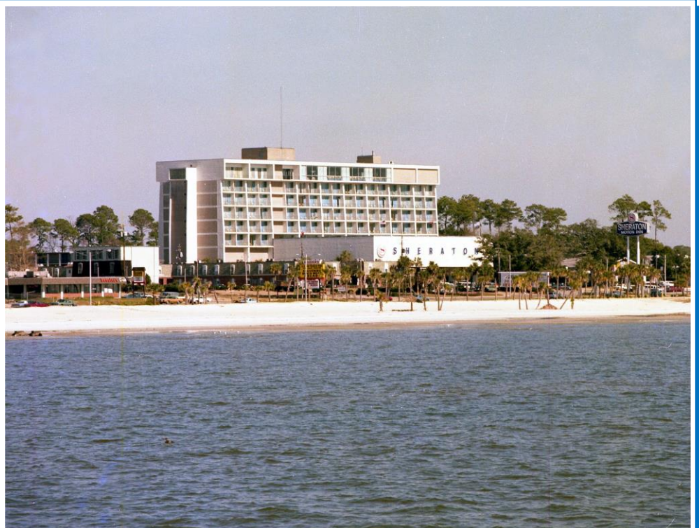
Biloxi's Treasure Bay Casino was originally called the Sheraton Biloxi Motor Inn. Ground breaking for this new 300 room hotel was held on March 6, 1969 (Thanks to Biloxi Library)
