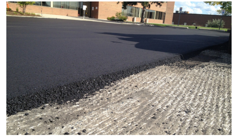
The milled surface is rough, but driveable, and is ready to be overlaid.
