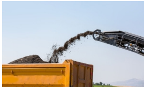
The old asphalt is passed through the mill-ing machine and fed into a dump truck.
