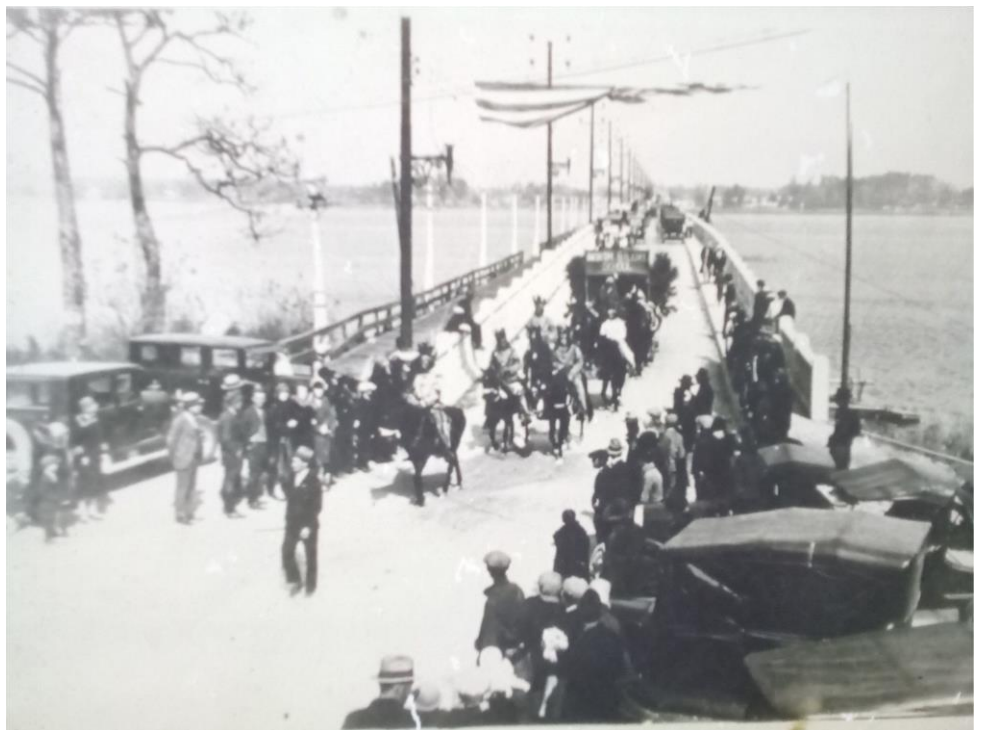
Biloxi Bridge (Back Bay bridge) that connected the north end of Caillavet Street (Biloxi) to Central Avenue (what's now D'Iberville), circa 1920s. The I-110 bridge was constructed west of this bridge in the mid-1970s.
