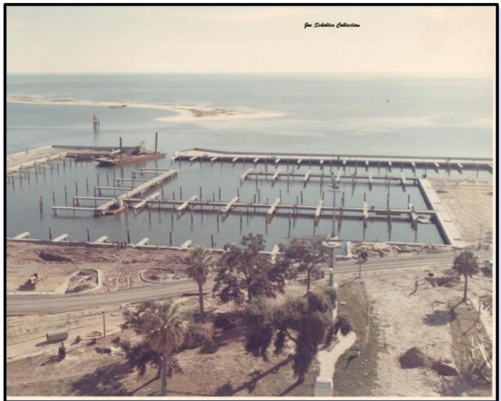
Biloxi Small Craft Harbor construction (Joe Scholtes Collection, No date)
