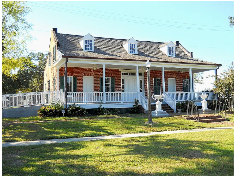
The Old Brick House, Bayview Avenue, view from the south, 2011.
