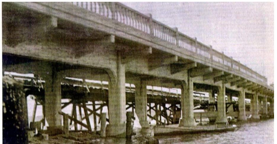
Original, wooden Biloxi Bay bridge built in 1901, and its concrete replacement built in 1926. Construction for the I-110 bridge to replace the concrete bridge began about 1973. This photo was taken in 1927.
