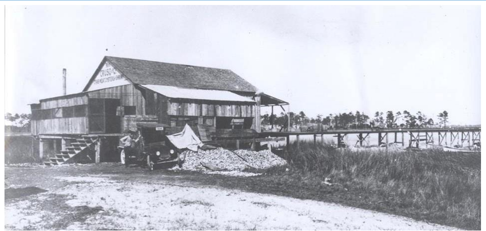
Bill Cruso's first seafood factory at Clay Point on Point Cadet; date unknown.
