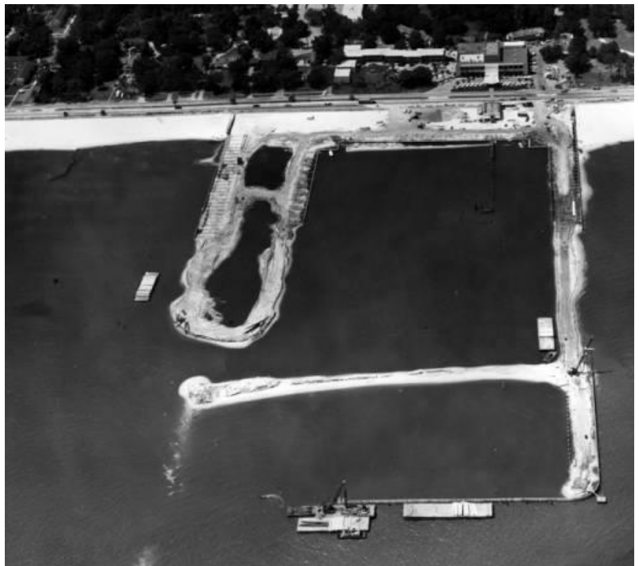
Broadwater Beach Marina under construction, Biloxi, circa 1964
