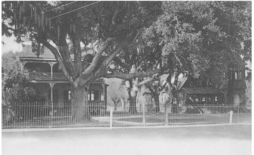
Episcopal Church of the Redeemer & Rectory, Hwy 90, Biloxi, circa 1940
