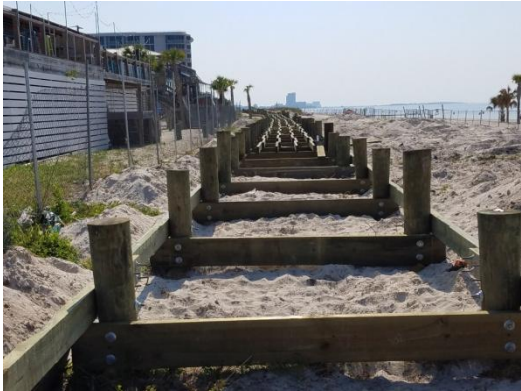
Boardwalk under construction, behind Bacchus restaurant, looking east, 05-13-18
