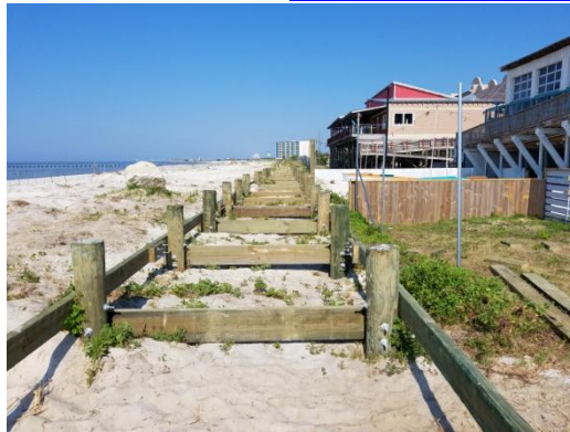
Boardwalk under construction, behind Bacchus restaurant, looking west, 05-13-18
