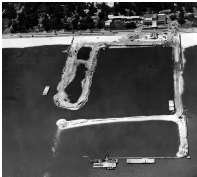
Broadwater Beach Marina under construction. Date unknown
