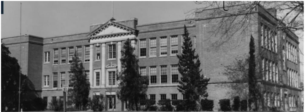
Howard II Elementary School, northeast corner of Howard Ave & Maple St. Destroyed by fire several weeks before Hurricane Katrina struck, 2005.
