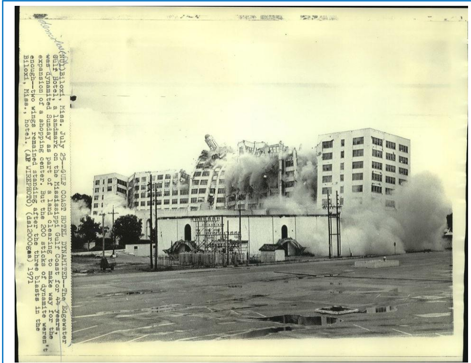
Demolition of the Edgewater Gulf Hotel, Biloxi, 1971, for the expansion of Edgewater Mall. This second demolition attempt proved successful.
