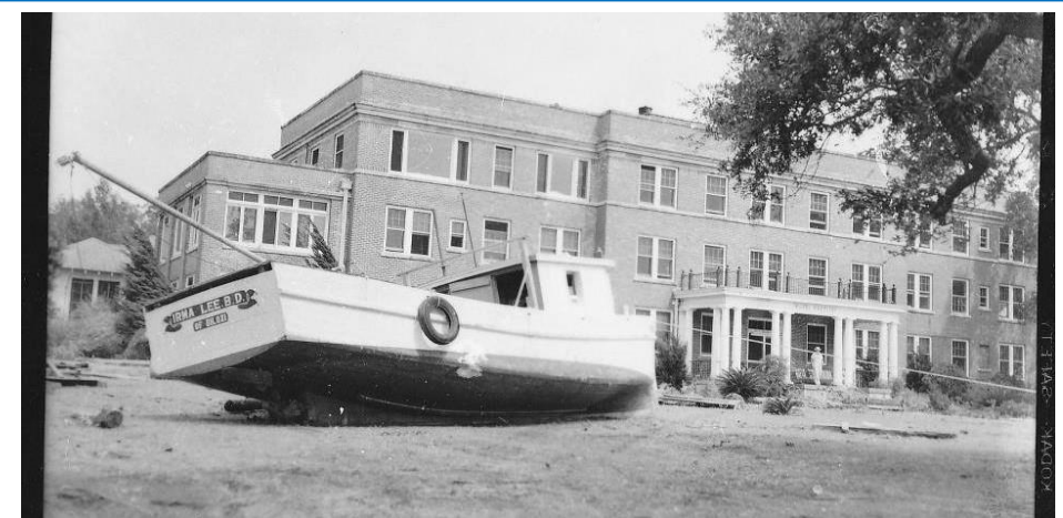
Biloxi Hospital, Highway 90, current site of the Hilton Garden Inn.
