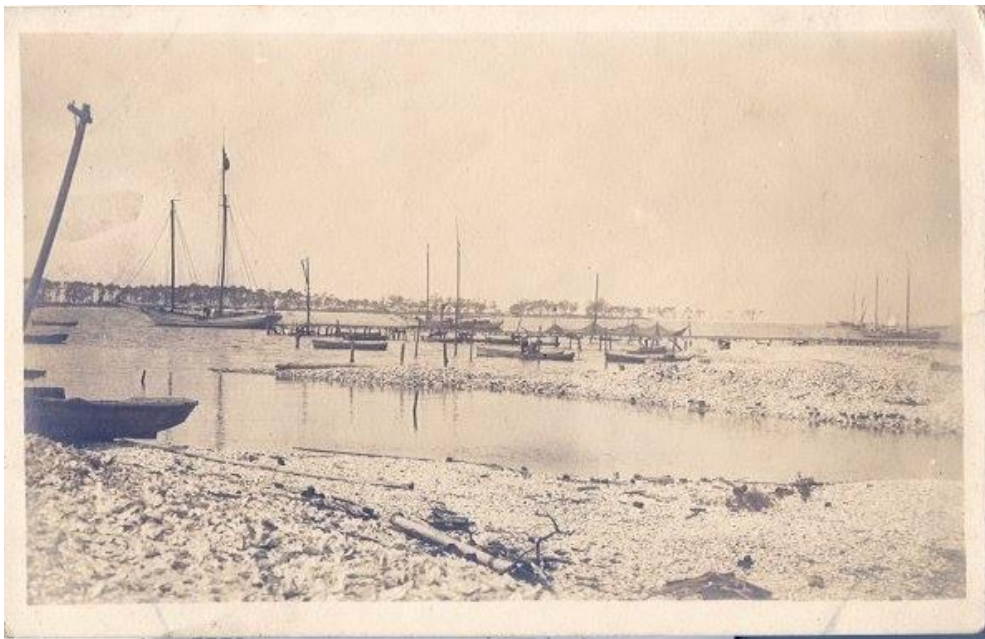
Biloxi beachfront, Deer Island in background, circa 1900 Oyster shells indicate a factory is nearby.
