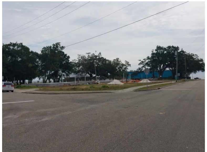
Apartments under construction, Briarfield Avenue
