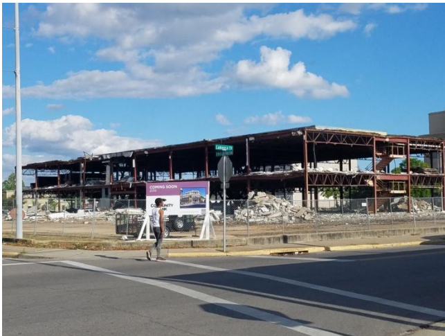
Demolition in progress, ole federal courthous
