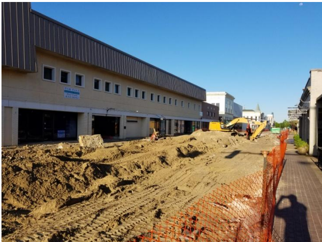
Howard Ave., looking east from Reynoir St.
