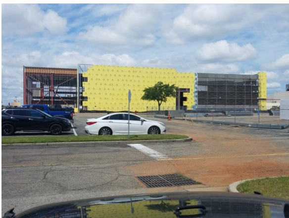
Eight screen movie theater at Edgewater Mall
