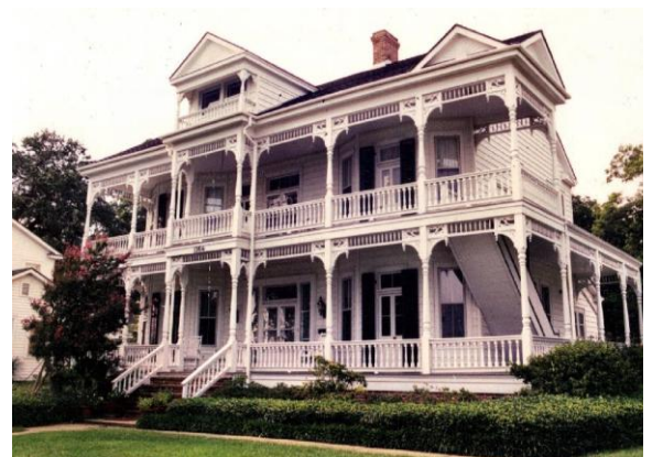
1364 West Beach Boulevard (Sutcliffe-Mavar); destroyed in Hurricane Katrina, 2005
