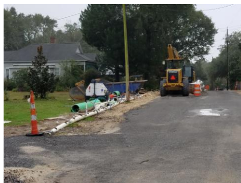
Water, sewer and drainage work continue south of the railroad tracks (Hemphill Construction) L to R: Father Ryan Avenue, Gill Avenue (looking south from Irish Hill) and Gill Avenue (looking north from Hwy 90)
