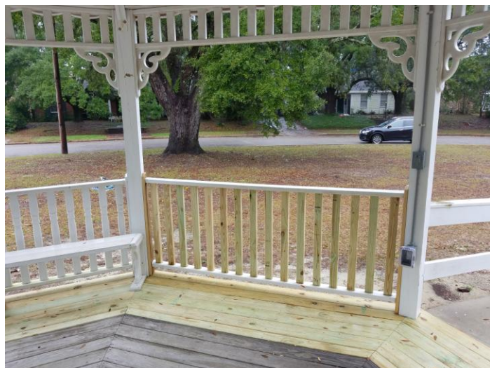
Edgewater Park gazebo repairs; painting this spring.
